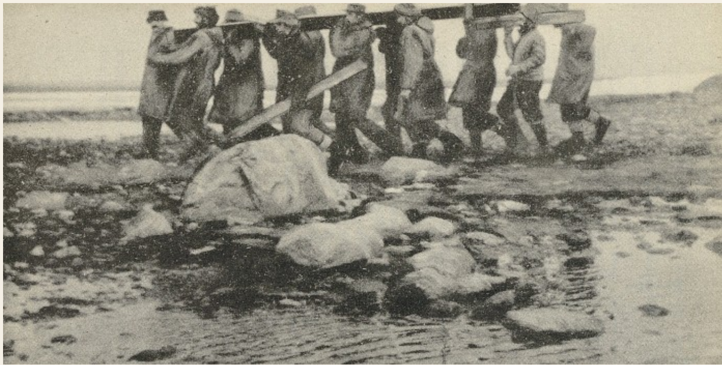
Hauling construction materials ashore.
