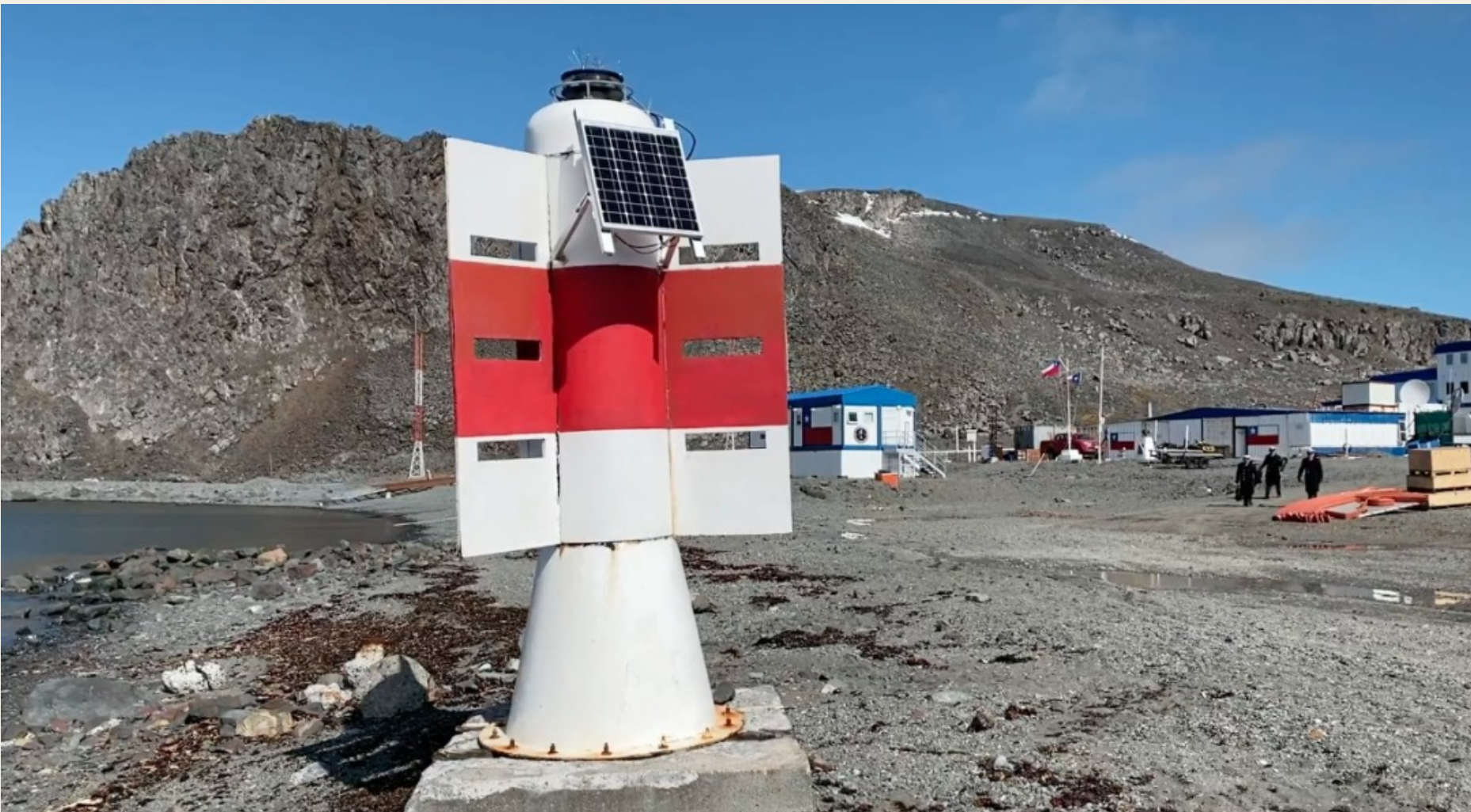
Solar-powered beacon with daymark boards beside a Chilean Antarctic base.
